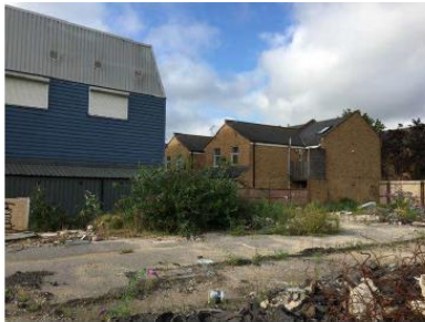
2. VIEW WITHIN SITE TO REAR OF ESIN COURT
