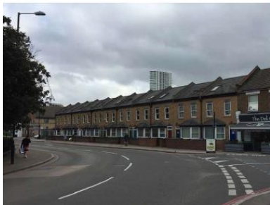
4. VIEW OF ESIN COURT FROM BROAD LANE FURTHER SOUTH
